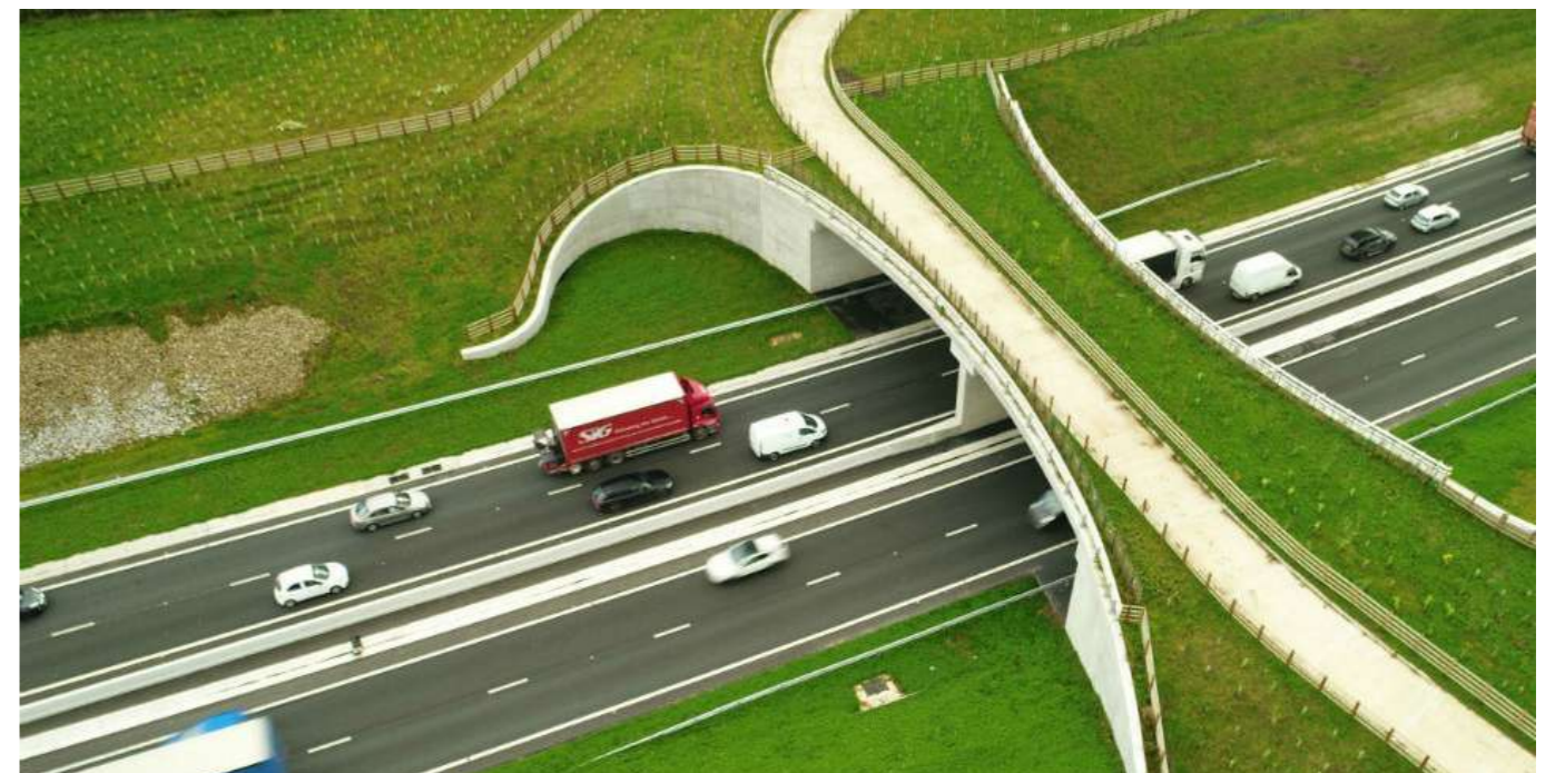
Figure 14: Photograph of an existing green bridge on A556, west of Mere (photograph courtesy of National Highways)
