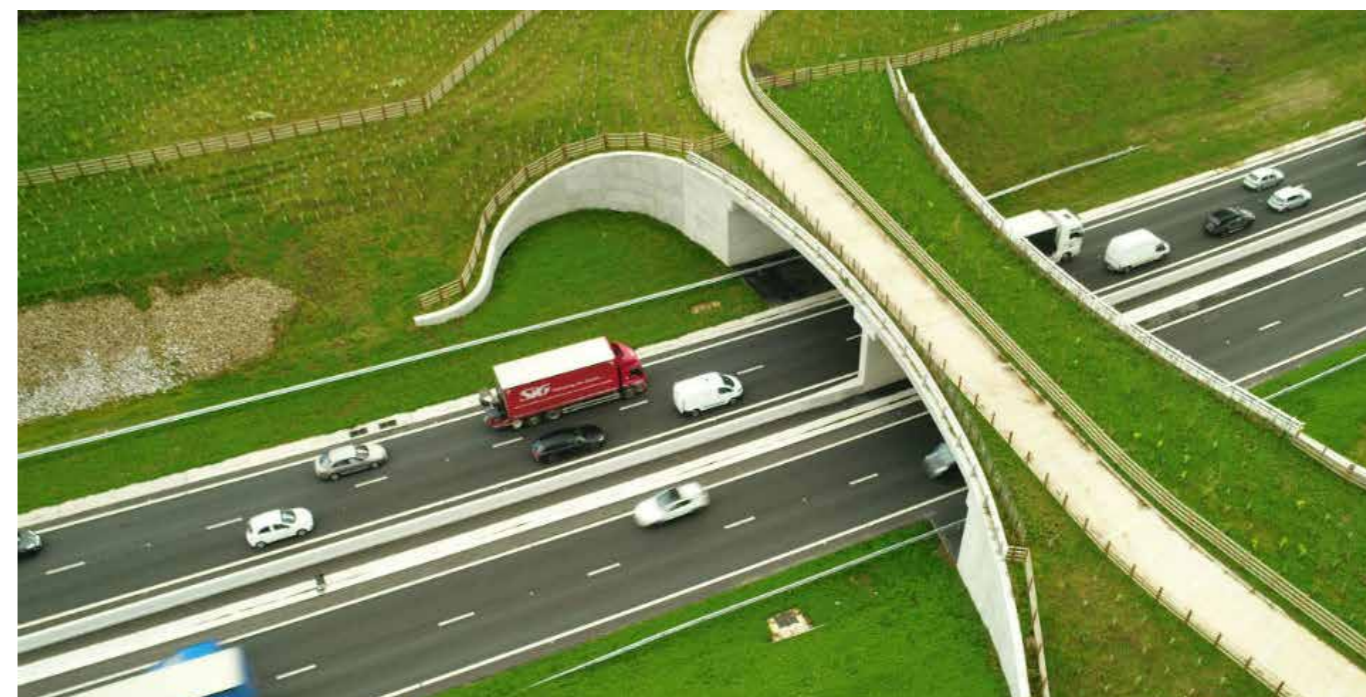
Figure 14: Photograph of an existing green bridge on A556, west of Mere (photograph courtesy of National Highways)
