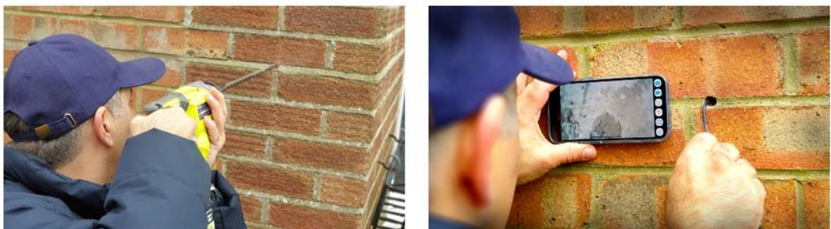
The photo above shows an example of an operative drilling a small hole in the mortar joint between bricks to insert a borescope camera. The image is then displayed and reviewed on site. We will repair the hole and the property will be returned to the condition it was in before the survey was carried out. Our team will avoid carrying out this work on any rendered walls.
