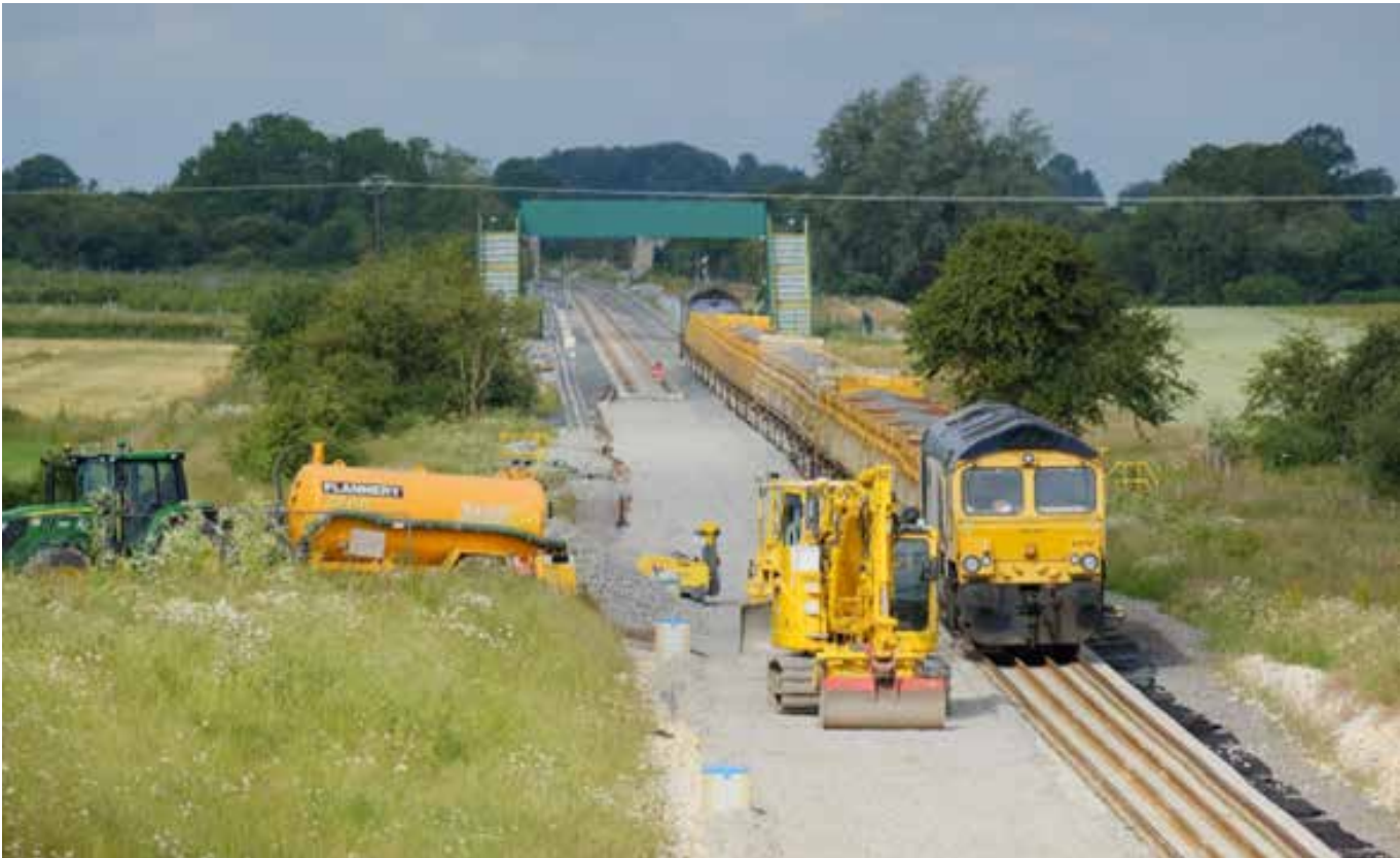
Figure 6: Construction works and track laying on Connection Stage 1 (Oxford to Milton Keynes)
